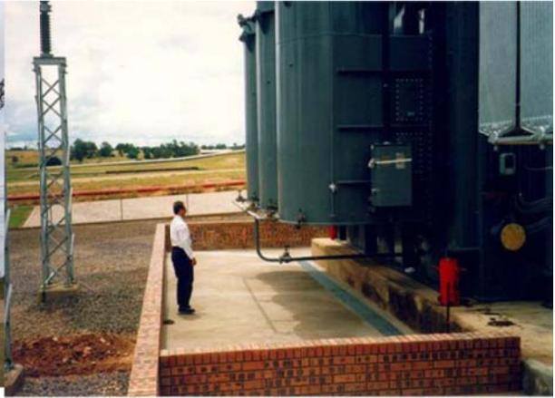
**Plate 2 - Transformer** approximate height 8m
