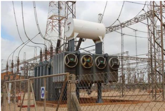
**Plate 3 - Transformer** showing oil reservoir and fans for cooling
