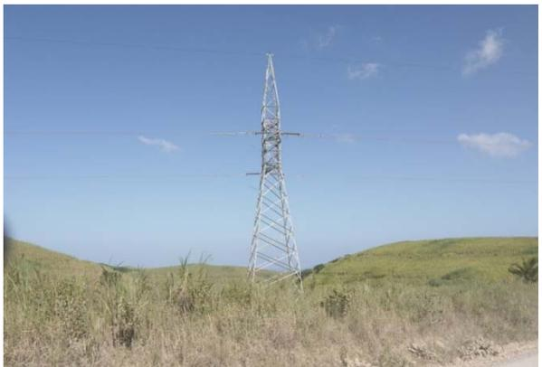
**Plate 6 - 132 kV Transmission Line Towers** 28m high
