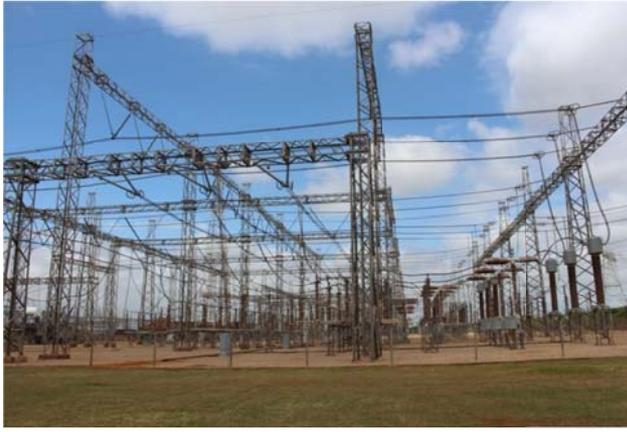
**Plate 1 - Sub-station Busbars** maximum height 22.5m
