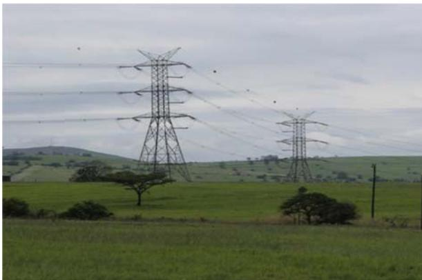
**Plate 5 - 400 kV Double Circuit Transmission Line Towers** 36m high
